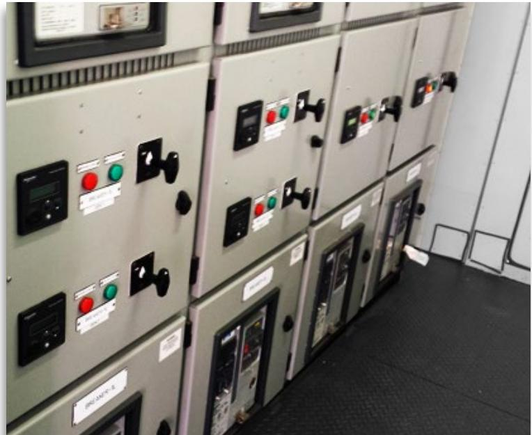
Paralleling SWG for 2MW Submarine Battery Charger
